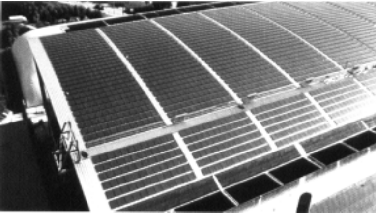
(Top) Figure I-2a. Roof-top photovoltaic panels will play a key role in on-site power generation. The natatorium of the Georgia Institute of Technology in Atlanta uses 32,750 square feet of solar panels. (Photo: Solar Design Associates)
